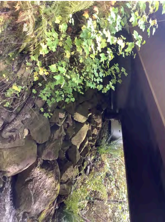
Left Bank Abutment when facing downstream
