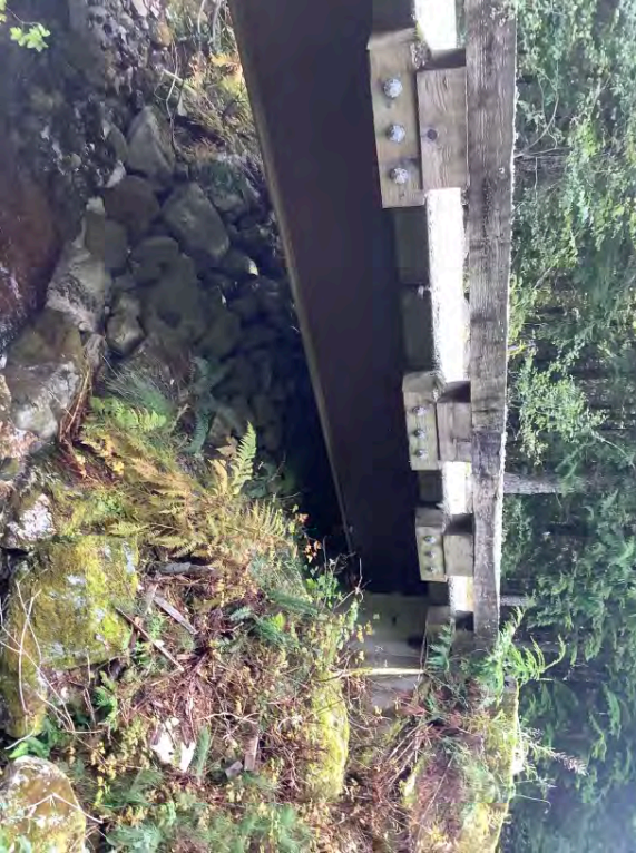
Right Bank Abutment when facing downstream
